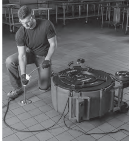
Figure 9 – Lubrification de la gaine de câble
